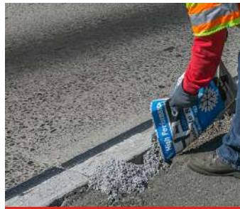
Fill Repair Area
