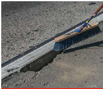
Clean Repair Area
