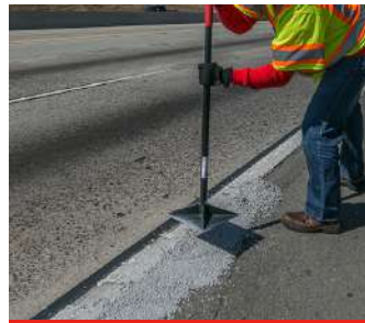
Tamp Repair Area
