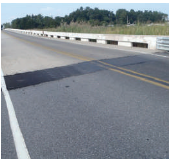
Bridge Deck Approach
