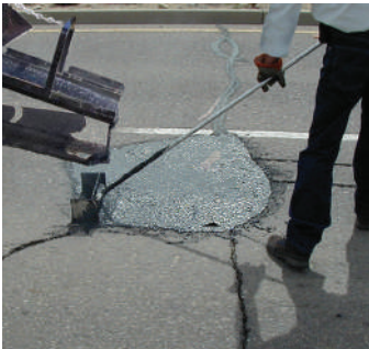
Pothole Repair
