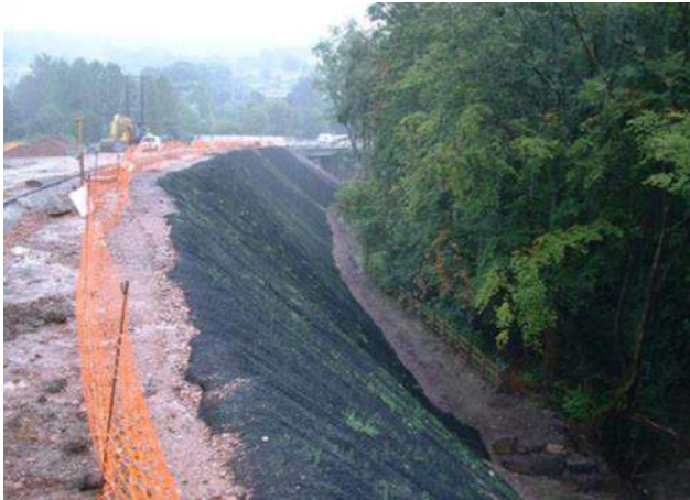
Erosion Control- Protecting slopes and waterways with Tensar Technology
