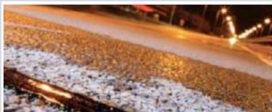
Joint, Crack and Patch Repairs
